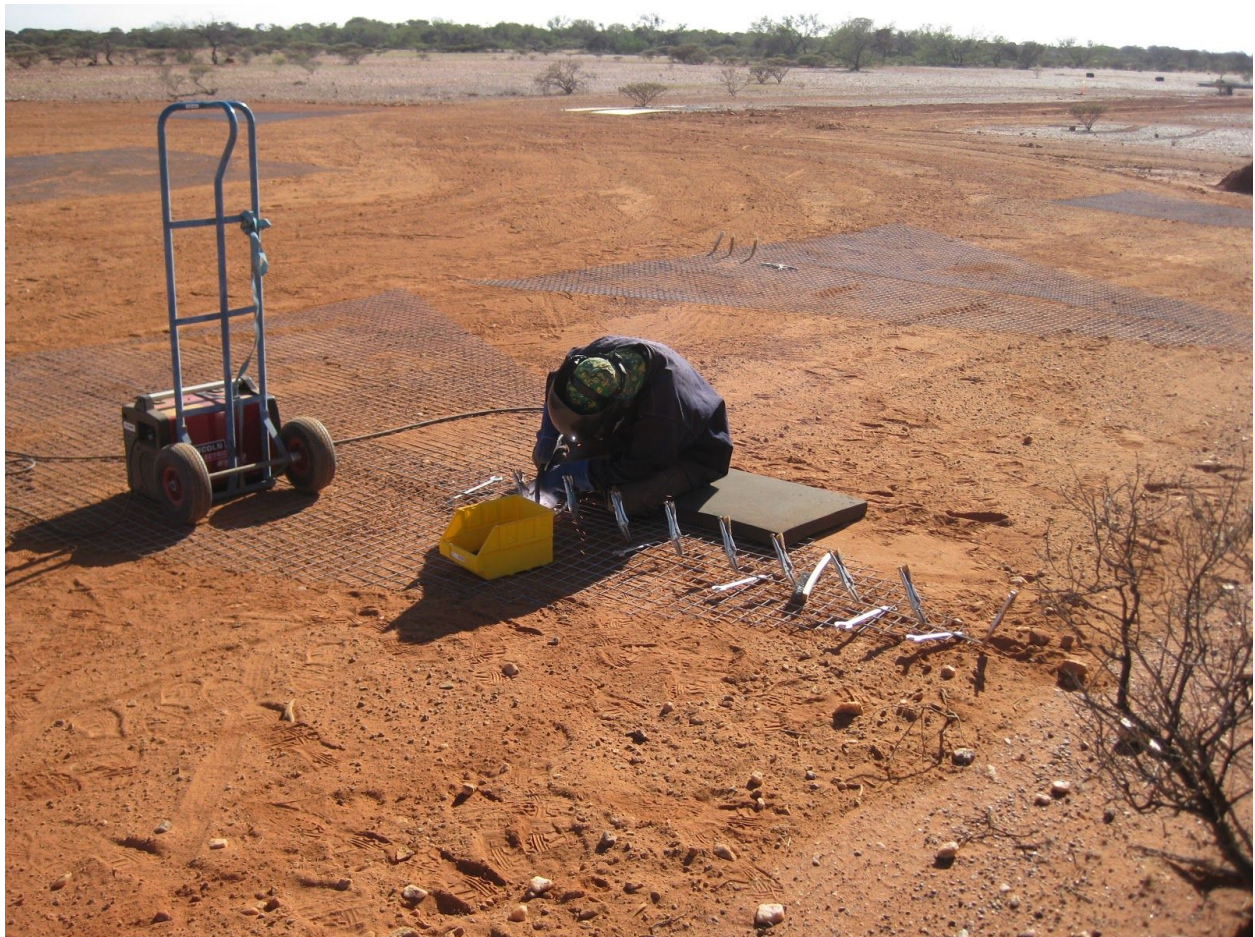
Figure 2. Welding set-up in March 2017.
